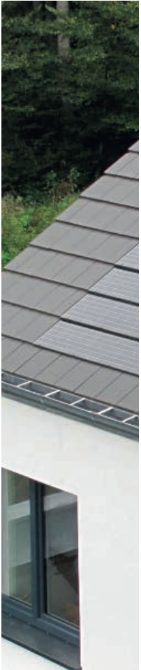
Solar Roof, Single-Family House Deining, Germany
